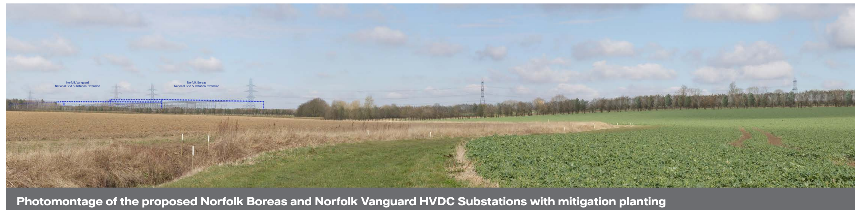
Photomontage of the proposed Norfolk Boreas and Norfolk Vanguard HVDC Substations with mitigation planting
